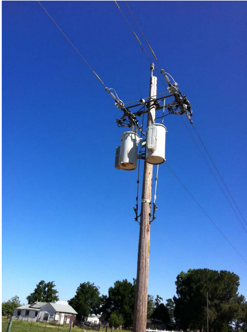
Figure 3-2: Open Delta Autotransformer 17/12 kV
